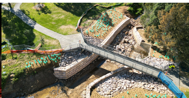
Burdett Street Footbridge Bank Stabilisation Works
