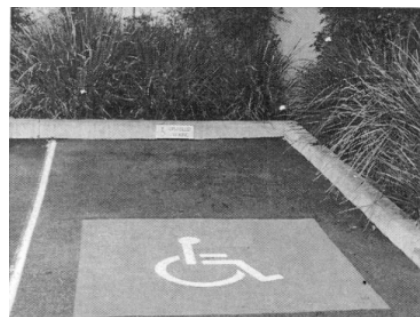
Figure 2 Disabled Parking Spaces are to be clearly identified through signage, logo and colouring
