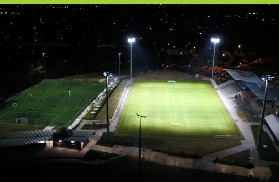
The elite field lighting at the Showground has been upgraded from 500lux to 1000lux.
