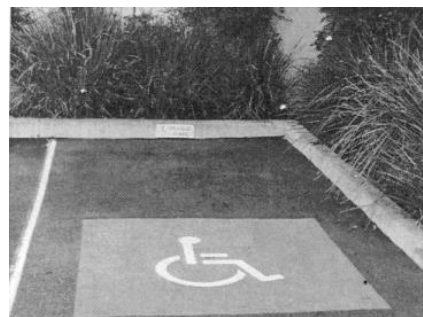
Figure 2 Disabled Parking Spaces are to be clearly identified through signage, logo and colouring
