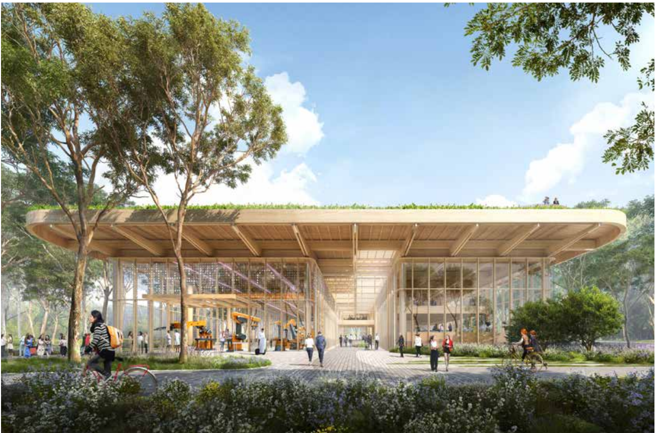
First Building housing the initial AMRF where a creative producer will be embedded. Image: Bradfield Development Authority.
