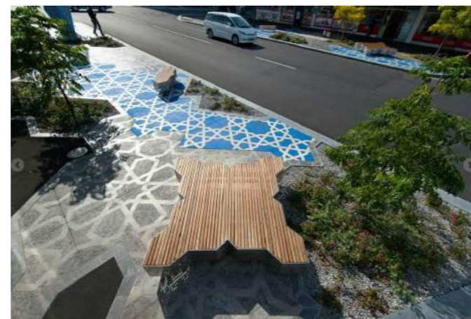
High quality streetscape treatments within large setbacks and plaza spaces in Villawood Town Centre to create a place for people (source Mark Wilson Media).
