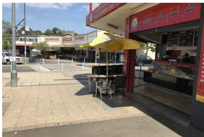
Building setbacks create a series of small plaza spaces along Villawood Place.
